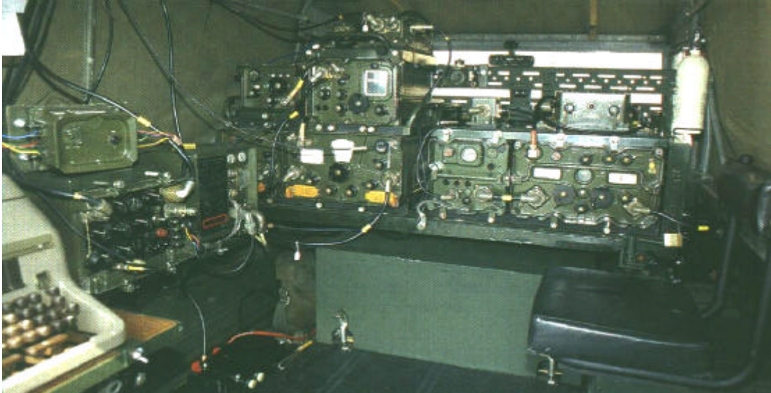
The Radio installation in Mick's Landrover. The T100 teleprinter can be seen on the extreme left.
