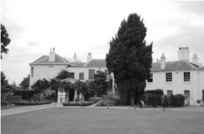
Fig.1 Pembroke lodge as it is today
